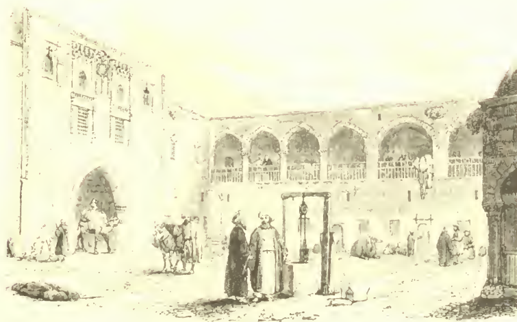
355 Interior of a Zir Khan, Aleppo. Frontal Drawing by E. Falkener, Esq.
