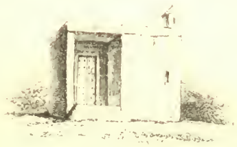
344] Hut of Greek peasant, formed of mud embedding sticks and straw. Valley of Canharus.—F. Howes. Lyons.
