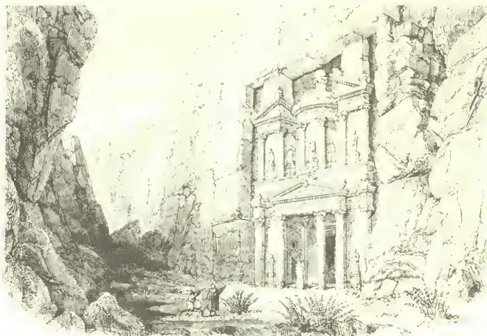
[354] Petra, South-east view of the Khasné.—Laborde.
