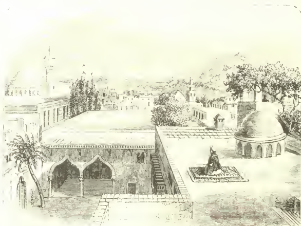
[343.] Flat-roofed Houses at Gaza. Laborde.
